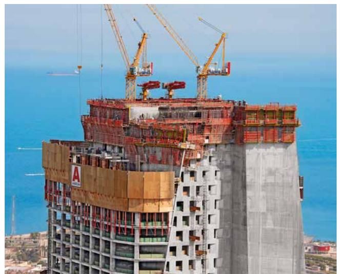
*PERI systems ensured that the exterior facades of the 412-meter-high Al Hamra Tower in Kuwait were protected during the manufacture of the floor slabs.*
